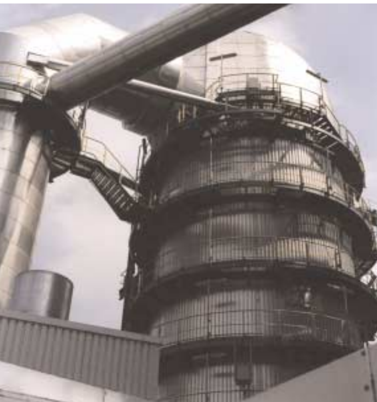
Flue Gas Desulfurization Unit “Chemische Werke Hüls, Germany” (Source: Krupp, Thyssen Nirosta)
