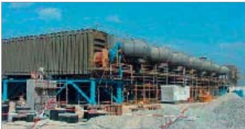
Figure 2. MSF installation nearing completion with water boxes connecting the various stages in the desalination process.
